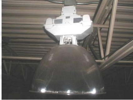
Old 250Watt Metal Halide Fixture w/lamp
