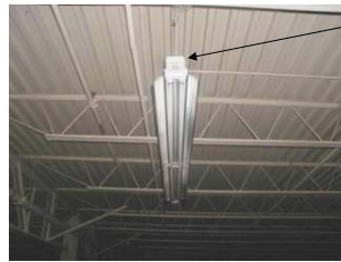
Aisle area lighting 2X2 T8's w/sensor 27
