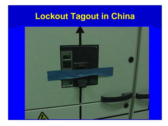
Scotch tape to prevent someone inadvertently flipping a switch—a 3<sup>rd</sup> party provider. 220 volt, no ground fault circuit breakers, live wire exposed
