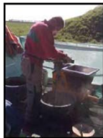
Mixing and applying Nanocrete mortar
